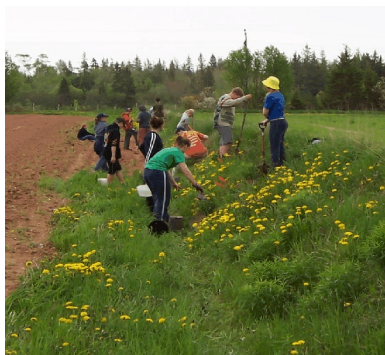
Planting shrubs and trees on diversion terrace
